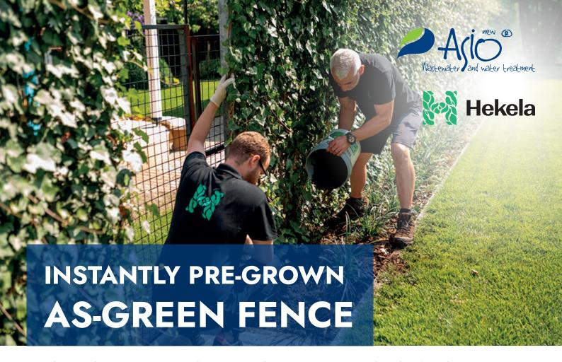
For those who want to enjoy the view of the greenery immediately after the construction is completed, ASIO brings the element of year-round green construction. The base is a zinc-coated structure with a width of 1.2 m and variable heights, greened with an undemanding climbing plant (Ivy - Hedera). Up to 5 individual plants are wound on each vertical bar. This ensures maximum coverage of the entire area.
