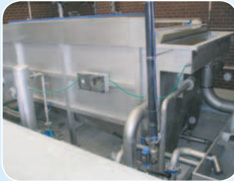
Placing of flotation unit AS-FLOT 100
