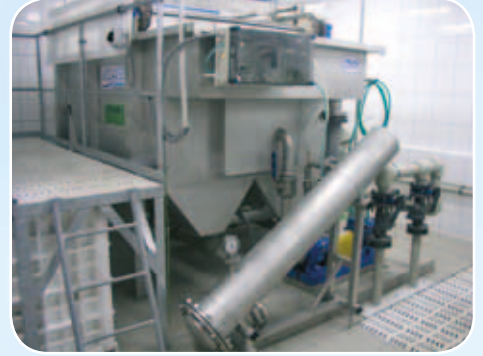
Placing of flotation unit AS-FLOT 10
