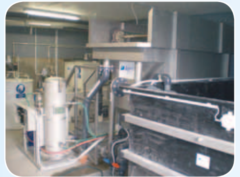
Placing of flotation unit AS-FLOT 3,6
