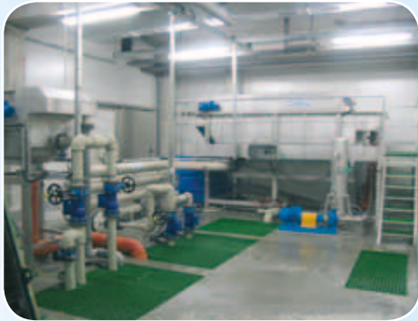
Placing of flotation unit AS-FLOT 40
