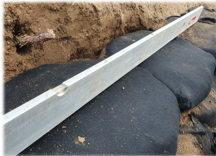
Checking the top row for flatness
