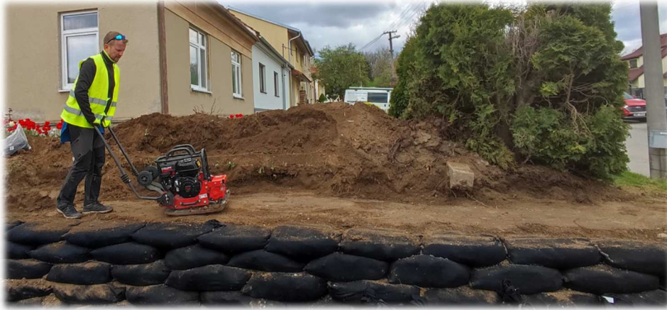
Compacting of layers by the vibration plate
