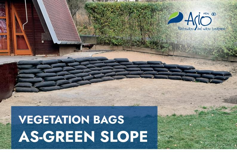
This is a system solution of stabilization of various slope types with vegetation bags, due to which it is easily possible to form a stable green slope. In order to bridge height differences or slope reinforcements, various concrete blocks or other masonry solutions are often used, but they are not ideal for their high bulk weight, minimum water penetration or low noise attenuation. AS-GREEN SLOPE vegetation bags represent an ideal alternative to these conventional solutions.
